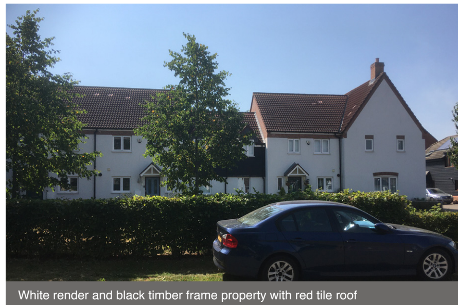
White render and black timber frame property with red tile roof
