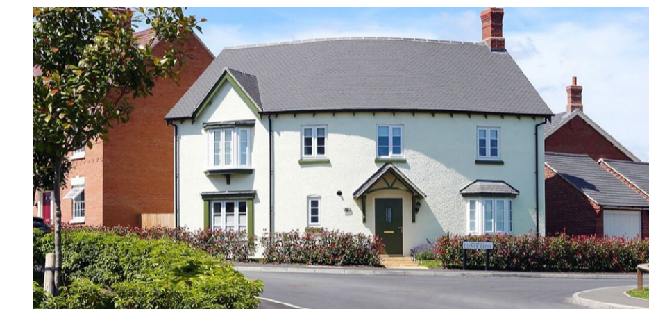
Corner unit providing active frontage and interest to the street
