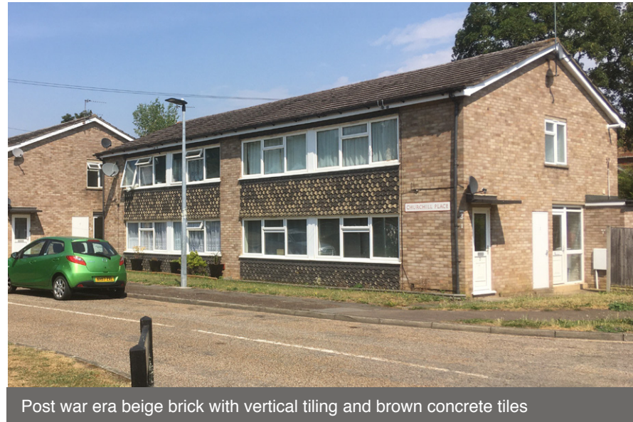
Post war era beige brick with vertical tiling and brown concrete tiles
