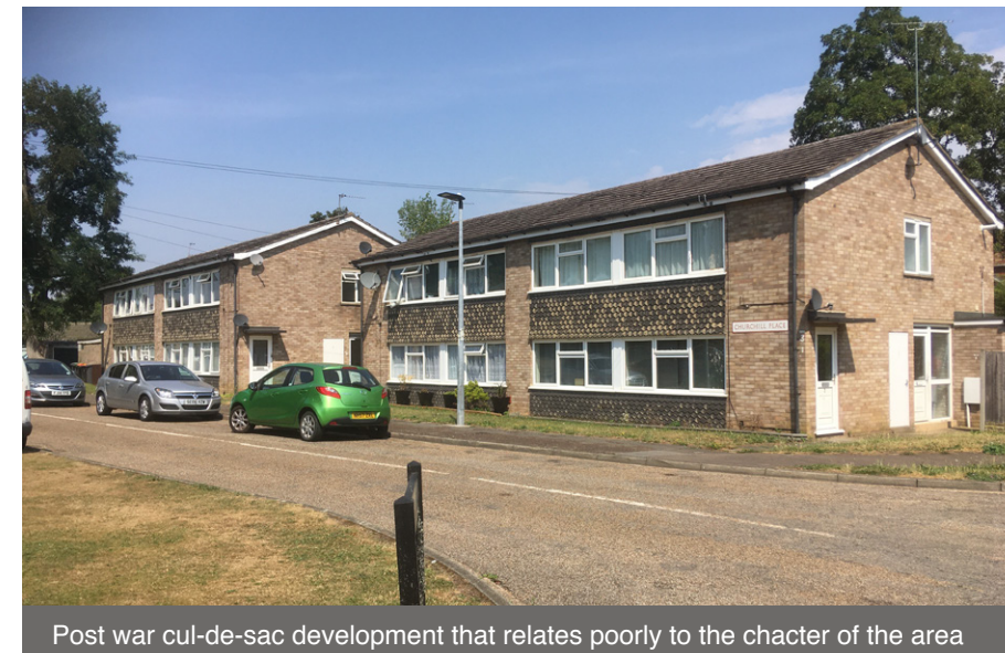
Post war cul-de-sac development that relates poorly to the character of the area
