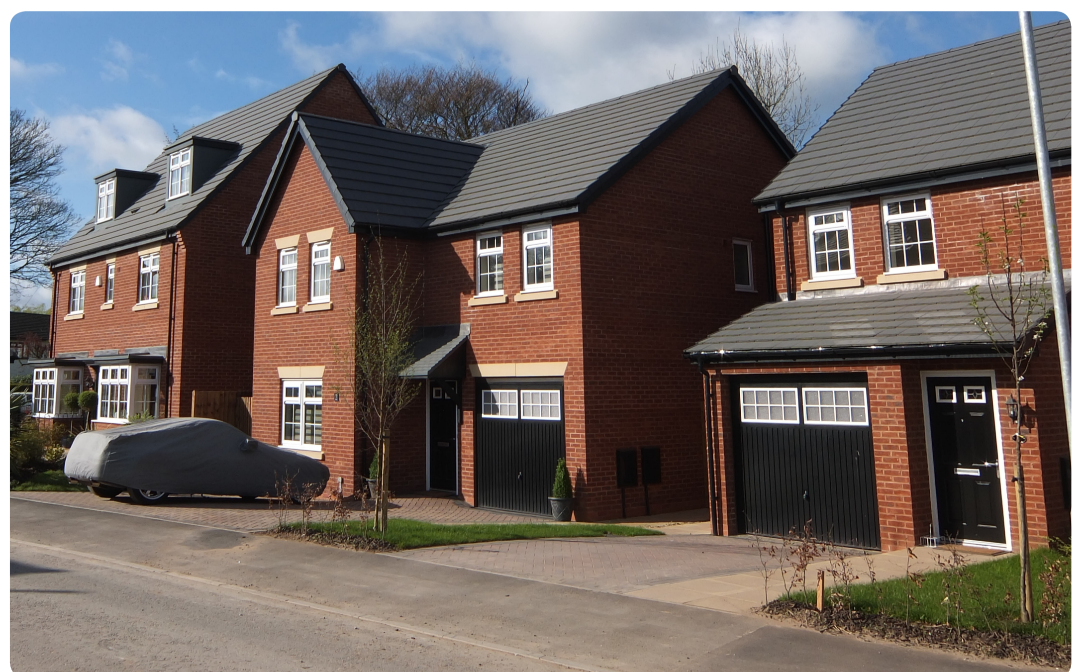
New housing at Monarchs Chase off Lightfoot Lane
